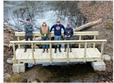
New bridge at Boulder Creek
